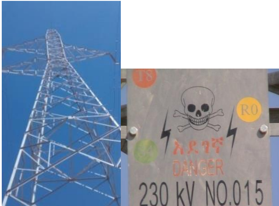
Fig. 6. The high-voltage pylon used for roosting by Alolobad
